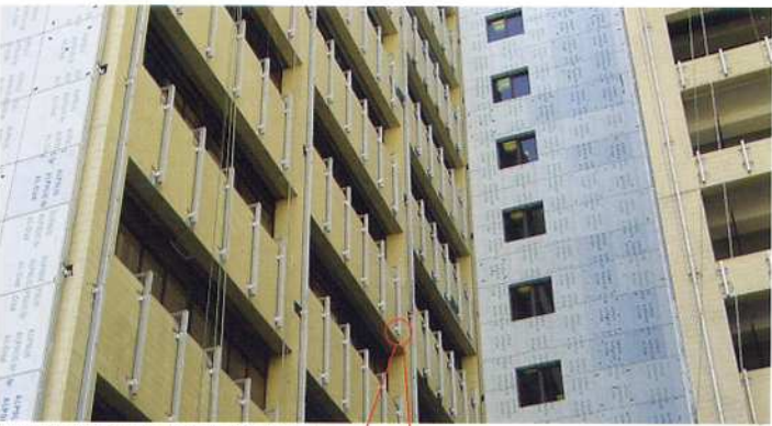
Mount Elizabeth Hospital & Medical Centre: before
