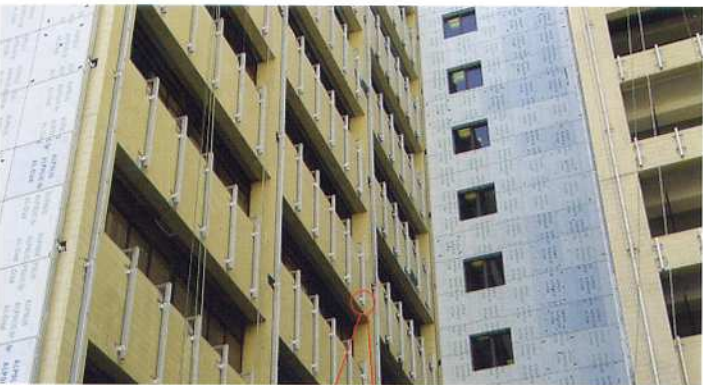
Mount Elizabeth Hospital & Medical Centre: before
