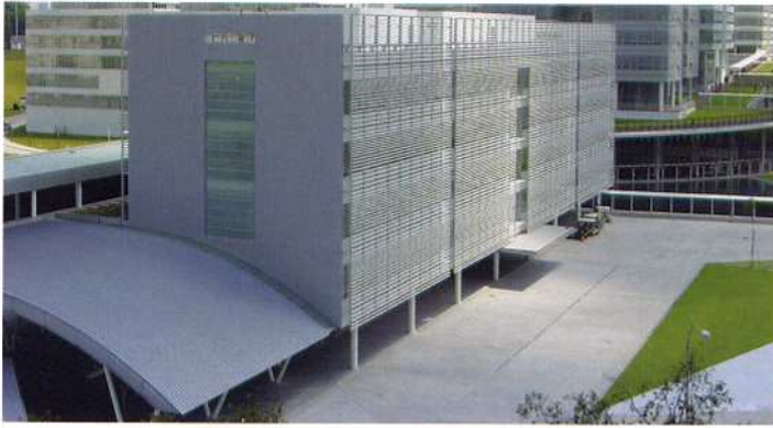
External cladding and steel structure were installed using Ramset anchors for Republic Polytechnic.
