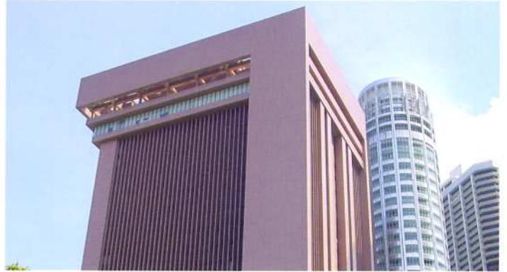
More than 100,000 pieces of stainless steel Ramset anchors were used for the external cladding of Monetary Authority of Singapore Building.
