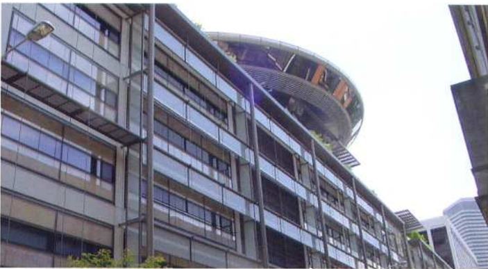
Ramset Anchors were used for the facade cladding of laminated marble glass veneer of The Supreme Court.
