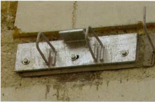
Main upgrading project using Split Triga Z for bracket of SAI
