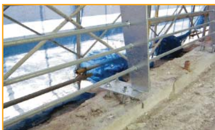
Installation of threaded stud for railing application.
