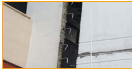
Installation of rebar component lapping to existing structure.
