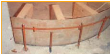
Anchoring starter bars for attachment of reinforcing for shower hob.
