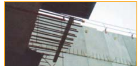
Anchoring starter bars to join vertical and horizontal elements.
