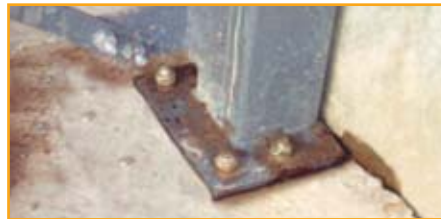
Close anchor spacing for structural steel.
