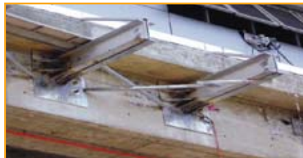
Installation of threaded studs for Cantilever.
