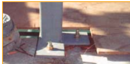
Permanent anchoring of steel columns to concrete floor slab.
