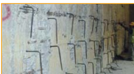
Rebar for skin wall construction in tunnel
